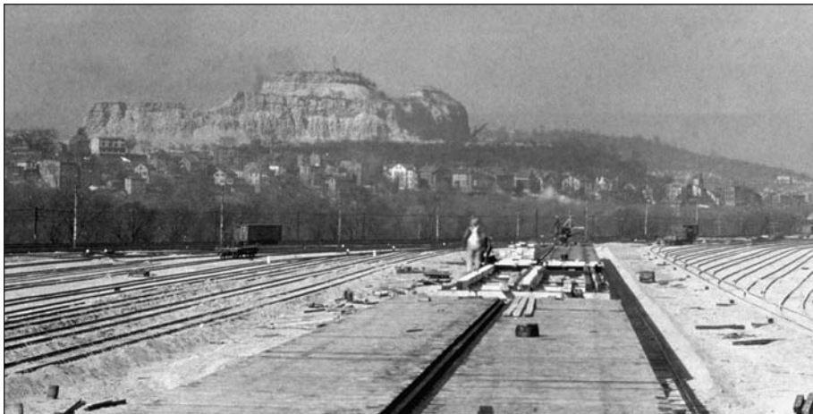
1930 photo showing construction of rail facilities at Cincinnati’s Union Terminal. Bald Knob is located in the middle background of the photo. This photo illustrates the extent to which mining and stripping of bedrock for fill material had impacted Bald Knob prior to and during the Union Terminal project. Photo from the University of Cincinnati archives.
