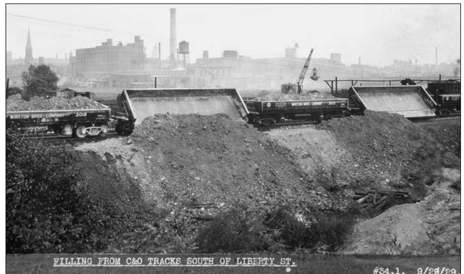
1930 photo showing construction of rail facilities at Cincinnati’s Union Terminal. Bald Knob is located in the middle background of the photo. This photo illustrates the extent to which mining and stripping of bedrock for fill material had impacted Bald Knob prior to and during the Union Terminal project. Photo from the University of Cincinnati archives.
